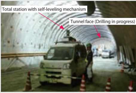
① Vehiclemounted measurement system in operation
