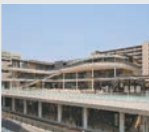
Belle Terrace Ikoma, Laurel Court Ikoma East Residence/ West Residence
