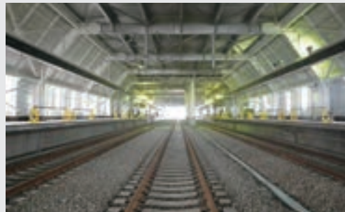
Oku Tsugaru Imabetsu Station of the Hokkaido Shinkansen, Oku Tsugaru Roadbed Work, Etc.
