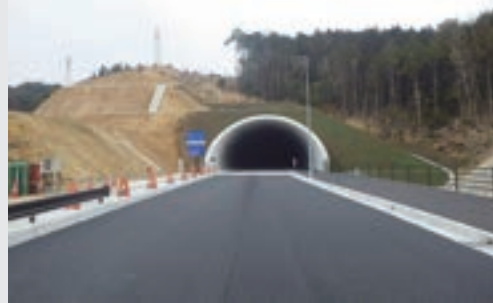
Maeyama Tunnel Work on Ochi Shirotori Bypass, National Route 11
