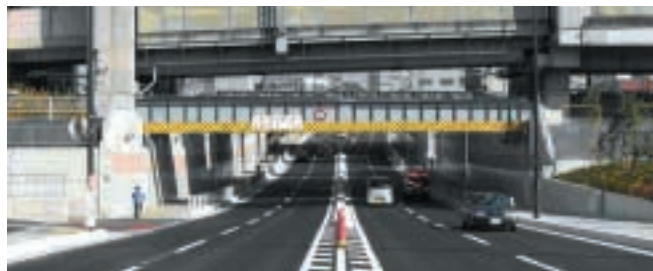
② Road reconstruction of the Second Yono Shindo Highway involving a two-level Intersection with the Tohoku Honsen Railroad in the Urawa-Omiya segment
