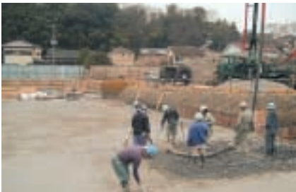
④ Placement of base slab
