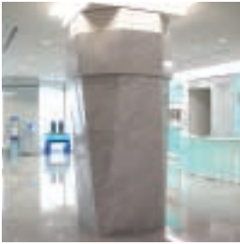
③ Column installed with a seismic isolation device
