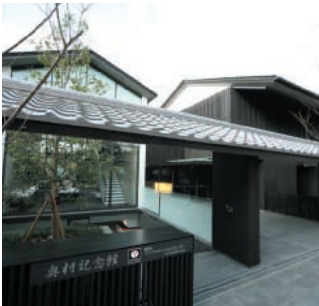
① Exterior view of the Okumura Commemorative Museum (seismic isolation structure)
