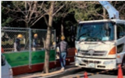
Fence installation work
