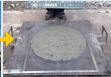
⑥ High-fluidity concrete (Slump flow 55 cm)
