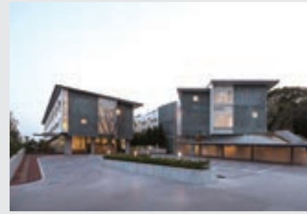
② Outside view of the Yahata Kousei Hospital Main Building
