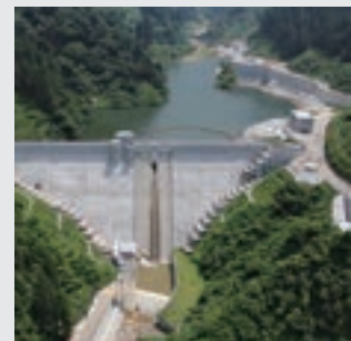
Funagawa Dam Construction in Funagawa Comprehensive Development Project
