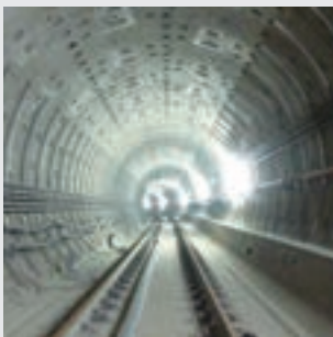
Work in Taoyuan International Airport MRT System Construction Project (Contract CU02A)
