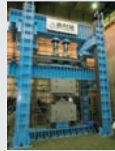
② Installation status of seismic isolation device
