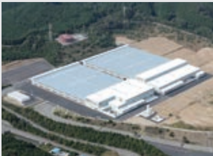
Kansai No. 3 Plant of SANKO Co., Ltd.
