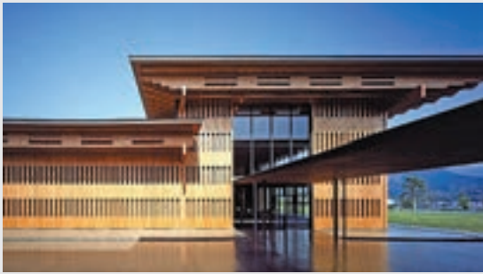
⑤ External view (connecting corridor)
