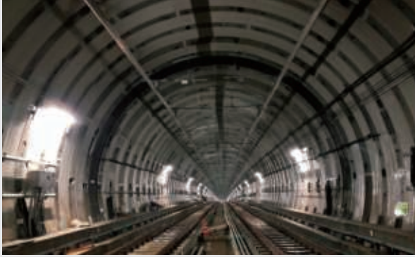
Sotetsu-Tokyu Link Line, Shin-Yokohama Tunnel
