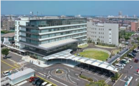
Kaizuka City Hall Work period: March 2020 to May 2023 Structure: Steel Total floor space: 12,351.4 m 2
