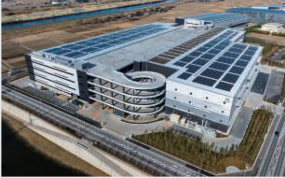
GLP ALFALINK Nagareyama 5 & 6 Work period: May 2021 to April 2023 Structure: PCaPC and partial steel Total floor space: 234,237.69 m 2
