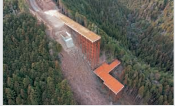
Substructure work for No. 7 Bridge, Shin Maruyama Dam National Route 418, Year 2021
