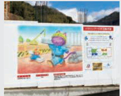
Hospital Construction Site (Hiroshima)
