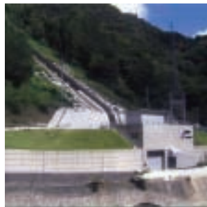
New Construction Project for the Shin-Taishakugawa Hydroelectric Power Station (Phase II)
