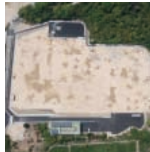
Kabutoyama Reservoir Construction Work
