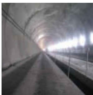
3: Tohoku Shinkansen Hakkoda Tunnel
