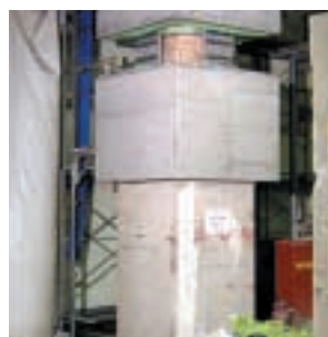
4: column with seismic isolation device installed
