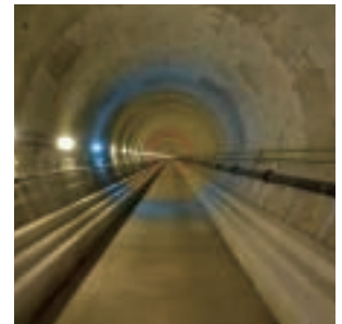
Civil Engineering Works in the Section of Takada B line of Tokyo Metro Subway line No.13
