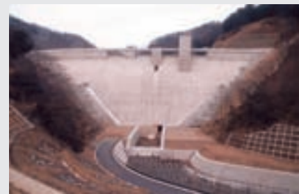
⑥ Flood-control dam construction at the Iwaigawa River
