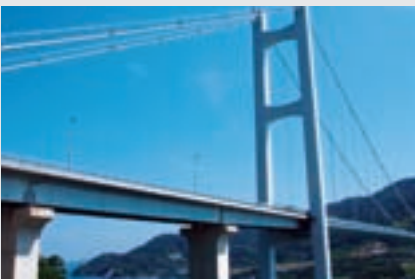
⑥ Toyoshima Ohashi Bridge
