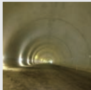
Hokkaido Odan Expressway: Tantaka Tunnel Construction Work
