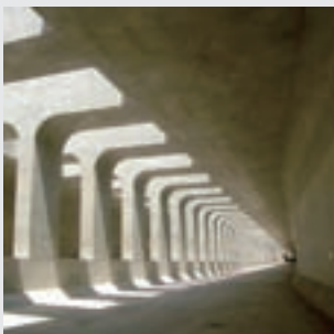
Higashi-Meihan Expressway: Shimada Construction Work
