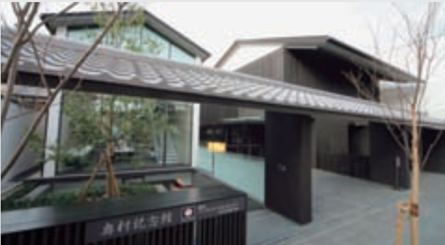
⑤ Exterior of the Okumura Commemorative Museum (seismic isolation structure)
