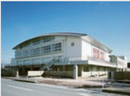
Kisarazu-Daiichi Elementary School: Feeding Center
